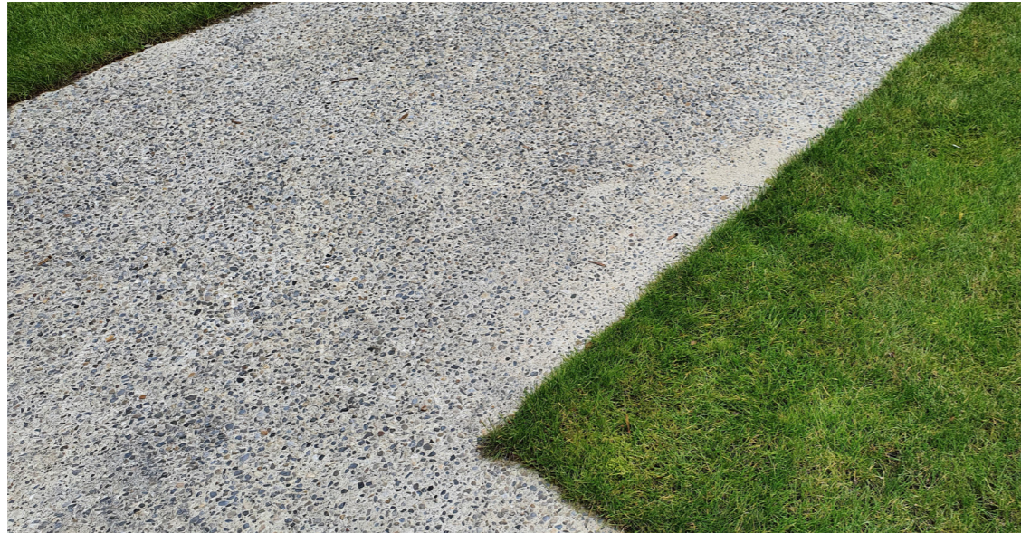
Exposed aggregate concrete footpaths
